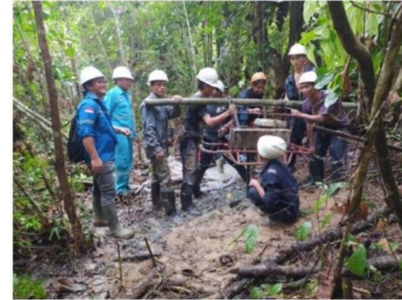
Shot hole drilling
