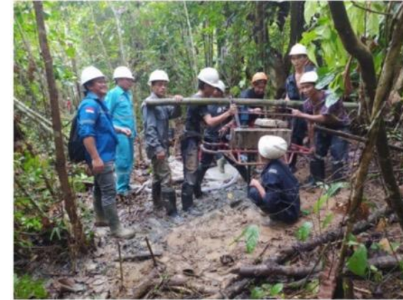
Shot hole drilling
